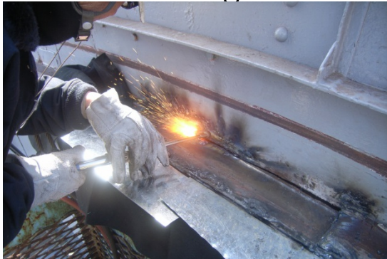
replacement of worn-out slit guide rail
