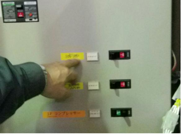
When the turbo pump reaches 0Hz, switch off the power behind the controller
