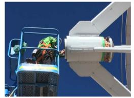
Manlift work is required to replace the malfunction motor
